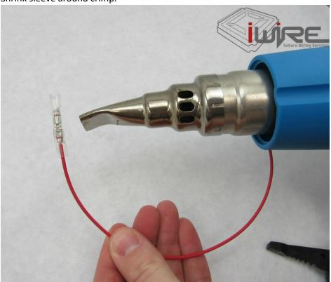
8. The shrink tube is fully recovered when you do not see any air bubbles and the glue comes slightly out of the bottom. After fully cooled redo pull test with moderate pressure.
